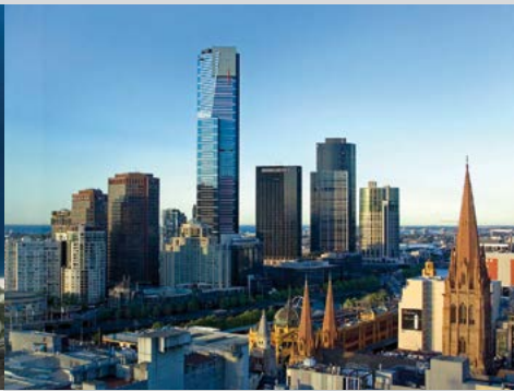
Eureka Tower MELBOURNE-AUSTRALIA
