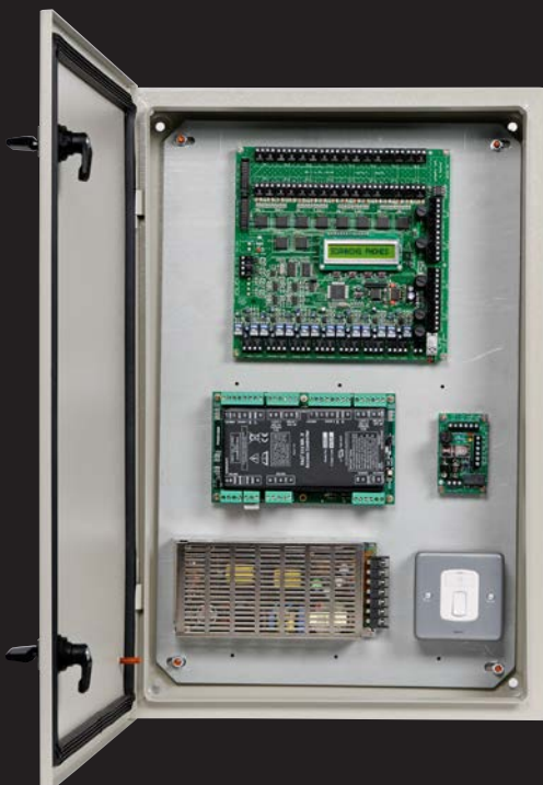
Typical GDX5 control rack with PAC controller fitted
