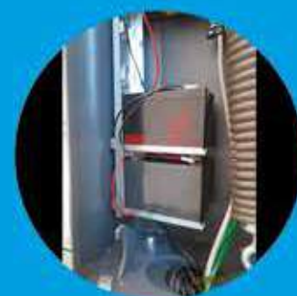
Emergency batteries
